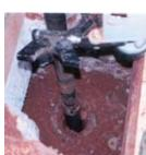
**Drilling through** shallow rock layer permits this Pre-Drilled Pier Bracket System to reach load-bearing stratum below.
