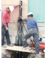
Installation by smooth hydraulic pressure extends pier to reach competent end-bearing soil stratum.
